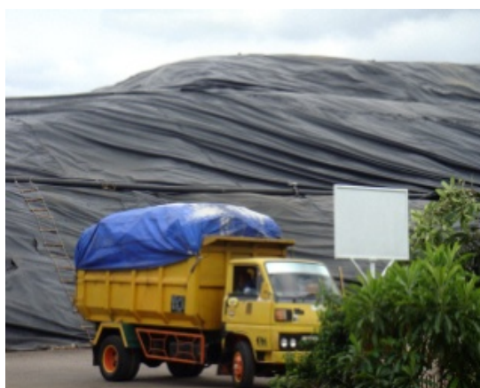
Figure 7. Landfill gas to energy generation
