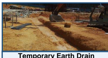
Temporary Earth Drain
