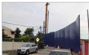
Temporary Noise Barriers
