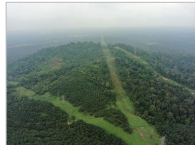
View of highest elevation (northern side)
