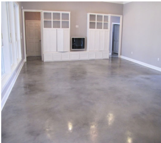
Fig. 8 Concrete flooring
