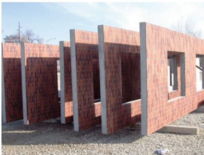
Fig. 6 Pre cast walls
