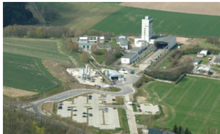
Fig. 6.8 Aerial photograph ERA Morsleben. Source BfS 2009
