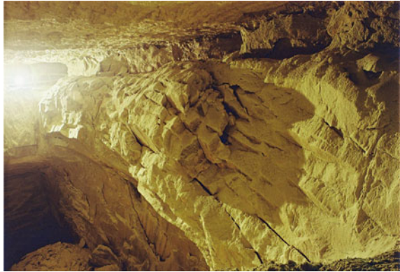
Fig. 6.19 Remains of a broken roof, mine workings row 7 south flank, photograph 2003. Source IfG [33]
