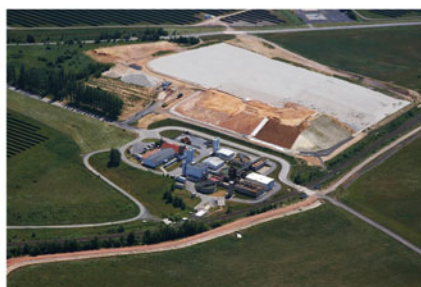
Fig. 6.4 Above: modified scheme of lime-Walhalla lime—water treatment process (WBA); [4]; bottom left: the storage field of the dump 371/1 with deposited big bags before sealing of the field; bottom right: Water treatment facility at Ronneburg. Source Figures bottom ©Wismut GmbH
