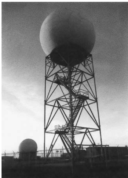
This geodesic radar housing protects the radar antenna. The whole system of which the housing and antenna are parts is called NEXRAD. The system incorporates the most advanced electronics and computer equipment. (Courtesy of the National Weather Service)
