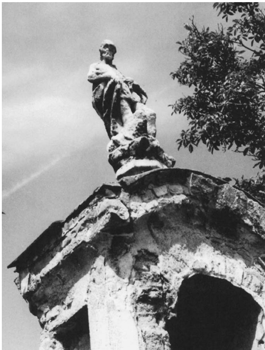
Acid rain attacks many materials. Limestone, a common material used by masons and sculptors, is particularly vulnerable. At one time, this limestone tomb was capped by a fine sculpture, but the stone has now eroded to a ruin. (Courtesy of Alexander Murashov, East Carolina University)
