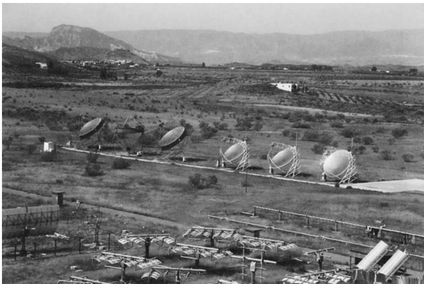
Each mirror in the array of cup-shaped mirrors automatically tracks the Sun and focuses the Sun's energy to heat water to makes steam. The steam is used to generate electricity. (Courtesy of the Sandia Laboratory, U.S. Department of Energy)
