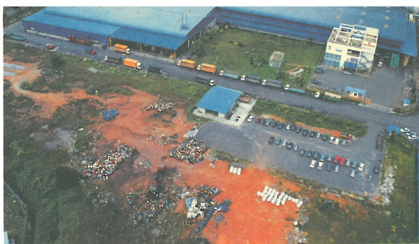
Photo 21 : Aerial view of Improper Scheduled Wastes Storage (DOE Photo Library)
