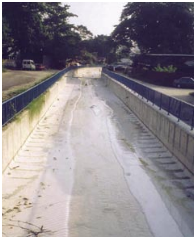
Polluted River : Cement Slurry from Construction Site (DOE Photo Library)
