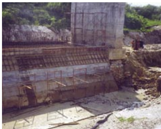
Polluted River : Construction Work Along River Bank (DOE Photo Library)
