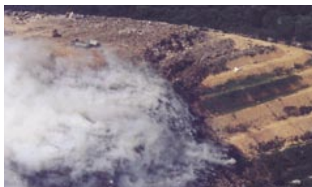
Aerial Photo of Open Burning at Municipal Solid Waste Disposal Site (DOE Photo Library)
