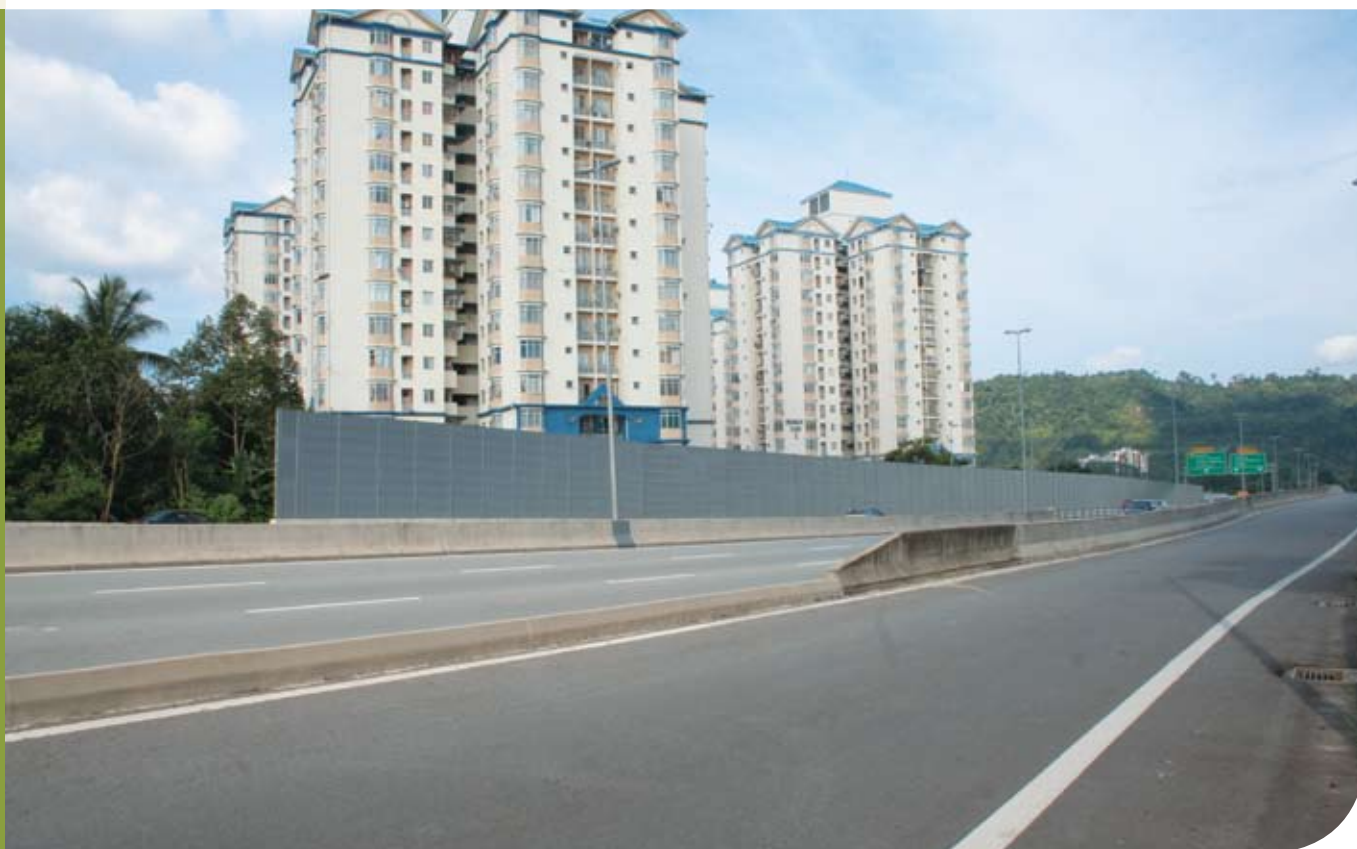
Noise isolating barrier walls installed along the highway
