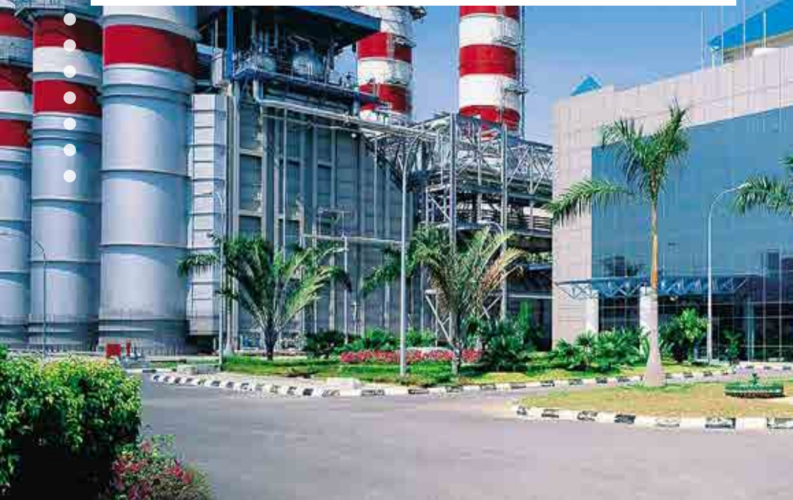
📍 Kuala Langat Power Plant, Selangor
