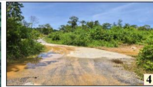
The main access to Project Site
