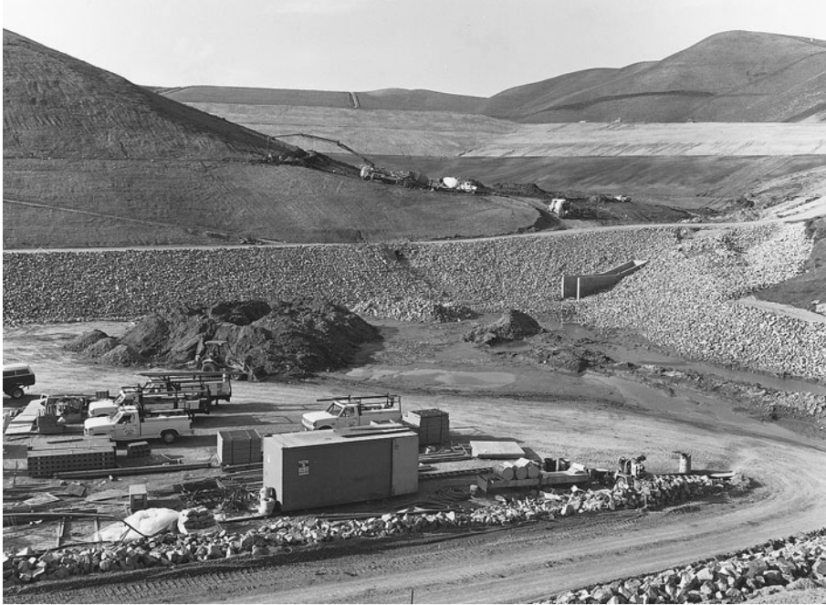
FIGURE 14.38 View of large storm water retention/storage basin at a large landfill. The size of the basin can be estimated from the size of the vehicles parked in the bottom of the basin.
