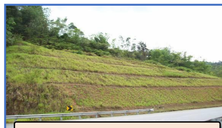
Example of Slope Turfing
