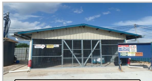
Scheduled Waste Storage Area
