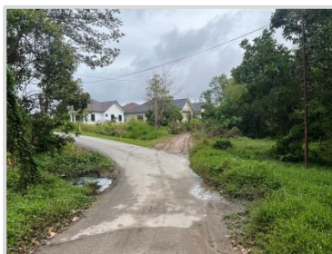
Road at the end of the Project alignment
