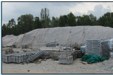
Example of Soil Stockpiles Covered with Geotextiles Sheet
