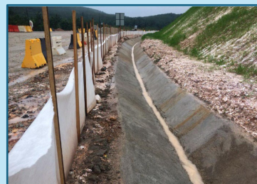
Silt Fence along Perimeter
