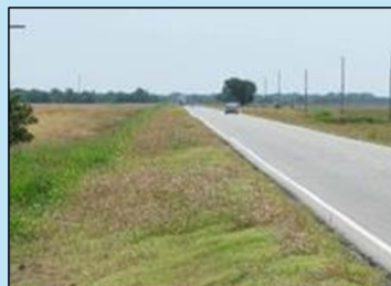
Example of Slope Protection
