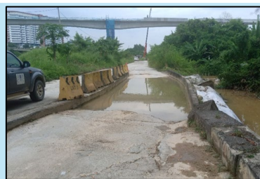
Example of Wash Trough at Site
