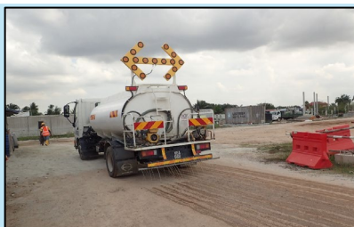
Example of Water Bowser Utilised at Site
