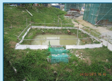
Example of Silt Trap
