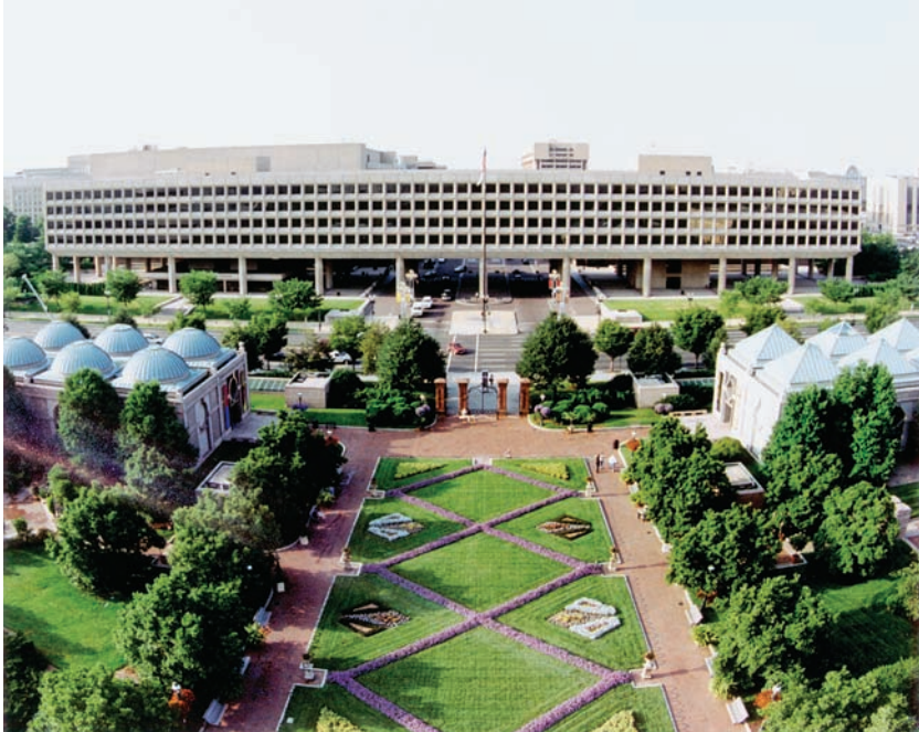
U.S. Department of Energy headquarters ( DOE )
