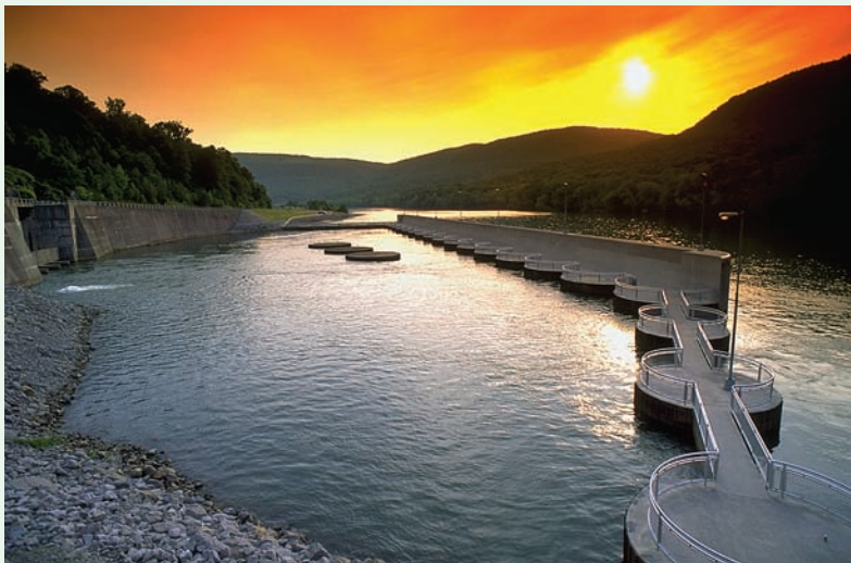
Tennessee Valley Authority pump storage facility, Raccoon Mountain (TVA)
