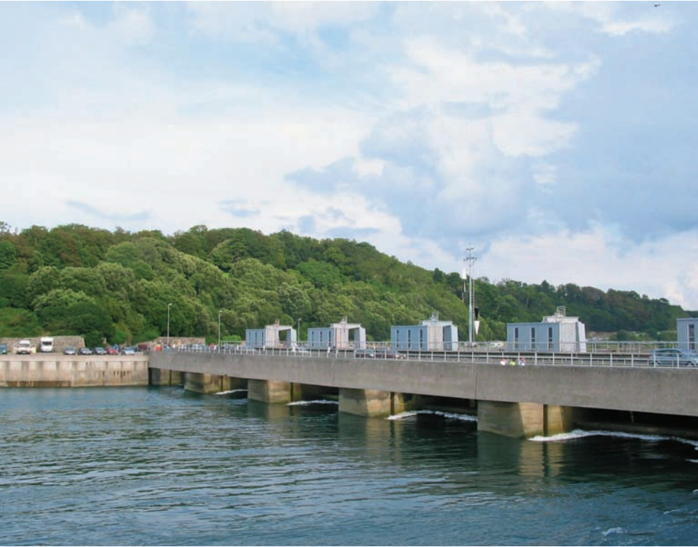
Part of the Rance tidal power plant in Brittany, France. Completed in 1967, it remains by far the largest facility of its kind. ( La Rance Tidal Power Plant )
