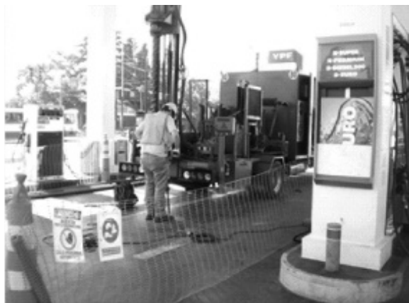
Figure 7.6 Drilling of injection well.
