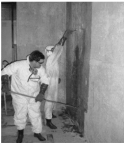
Figure 7.3 Application of nZVI slurry.
