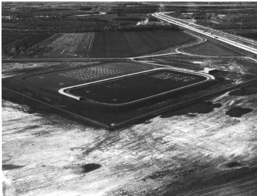
Fig. 6.12. Mixing patterns produced by air guns in an aerated lagoon treating municipal and food processing wastes (courtesy Aero-Hydraulics Corp.).
