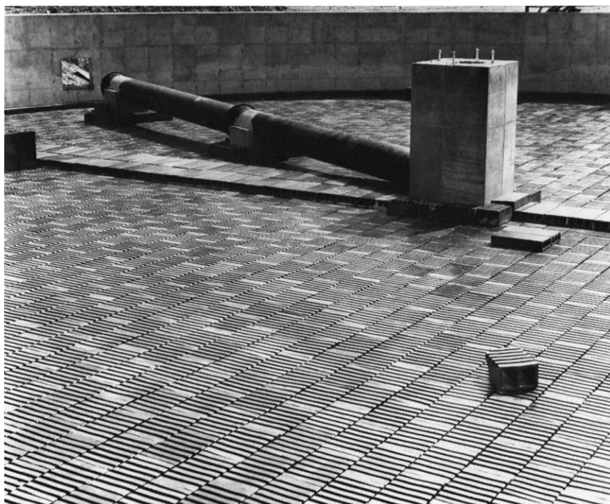
Fig. 7.28. Clay tile underdrain system for a rock media trickling filter. The influent pipe and riser to the rotary distributor is shown (courtesy W. S. Dickey Clay Mfg. Co.).
