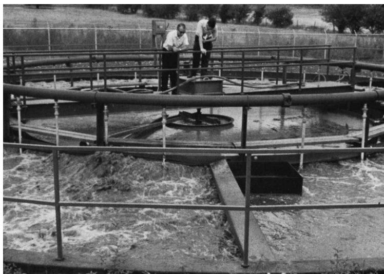
Fig. 7.14. A contact stabilization plant treating combined municipal and cheese plant wastes. The sedimentation section is in the middle with the contact and reaeration basins on the periphery of the circular unit.
