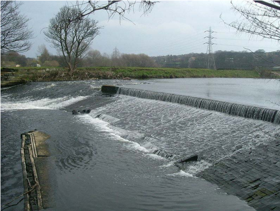
A weir on the River Calder, West Yorkshire
