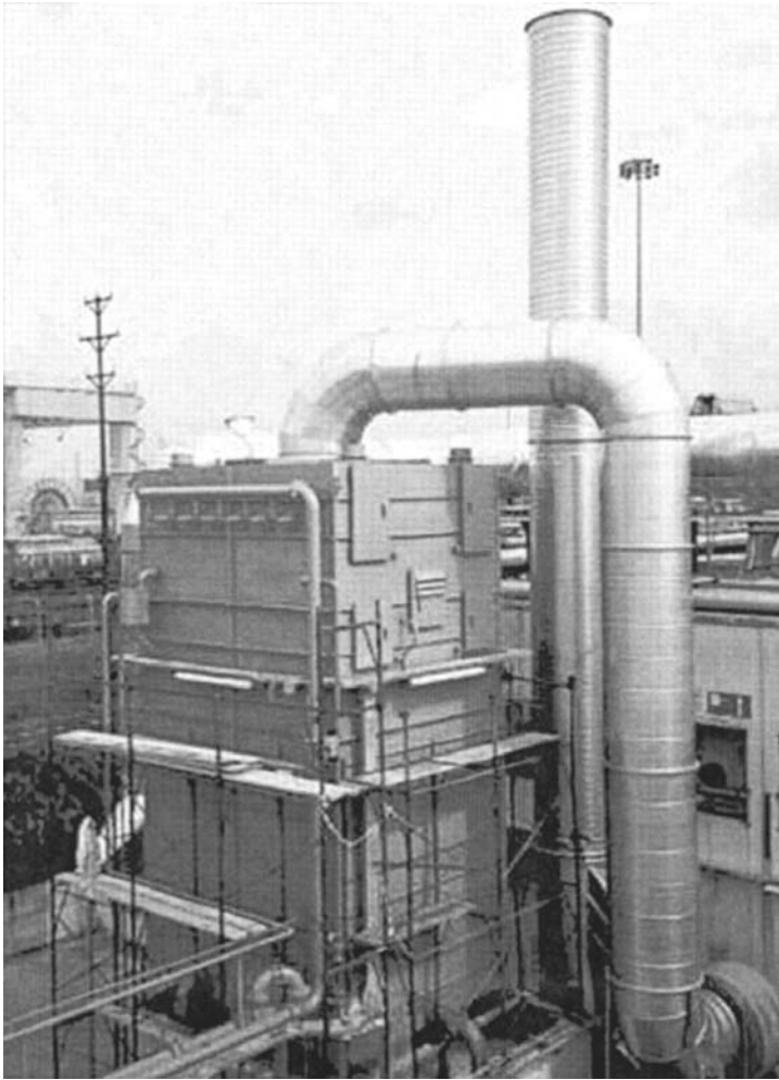
Figure 9.21 Industrial wet electrostatic precipitator. (Courtesy of Croll.)
