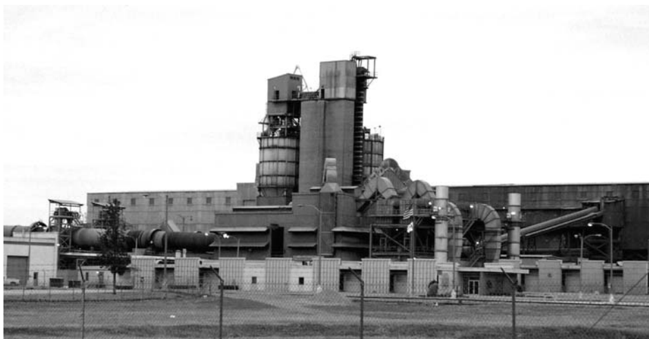
Figure 1.23 Cement manufacturing plant.
