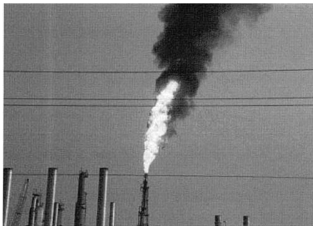
Figure 15.30 Typical elevated single-point flare. (From Ref. 63. Courtesy of John Zink Co. LLC.)
