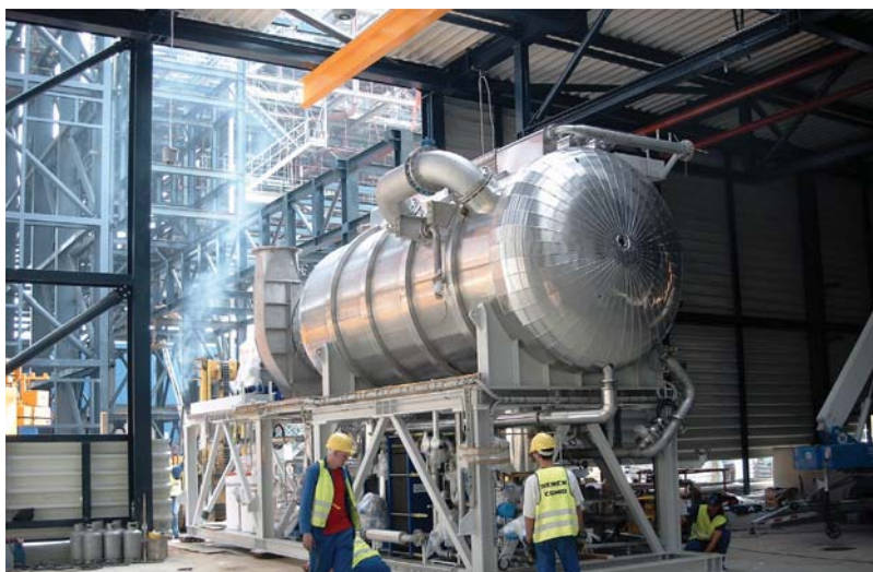
Figure 2.54 300 t/d - MVC evaporator during installation in a power plant (by courtesy of Hamworthy Serck Como GmbH, Geesthacht, Germany) [16].
