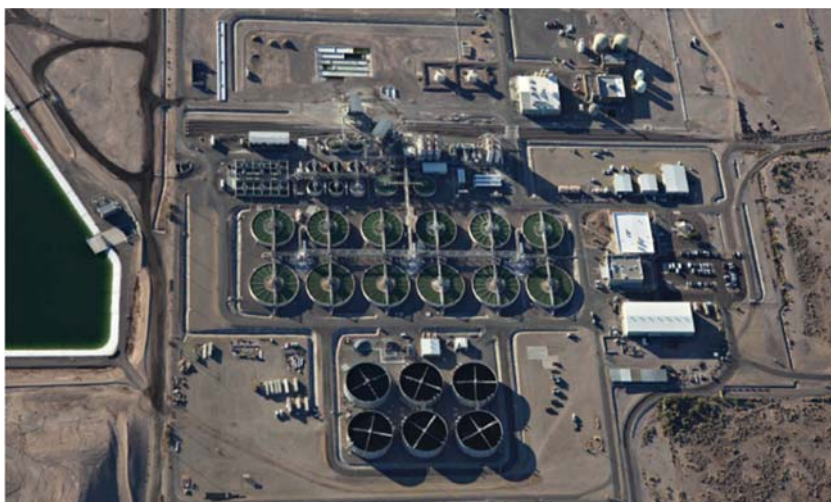
Figure 14.10 Palo Verde Water Treatment Plant (from Lott 2011).
