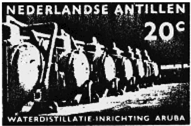
Figure 2.52 Multiple-effect seawater desalination plant on Aruba (1959)[13].
