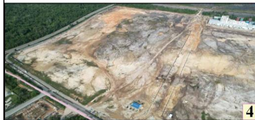
Overall view of the Project site from Southwestern Boundary
