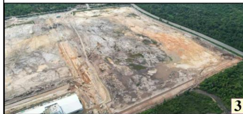
Overall view of the Project site from the Southeastern Boundary
