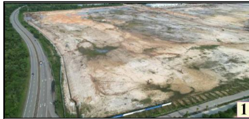
Overall view of the Project Site from the Northwestern Boundary
