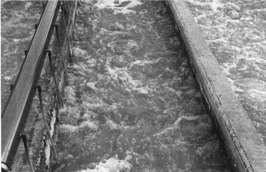
Figure 5.23 Photo of the SND pilot-plant at Vantinge on the island of Fyen.
