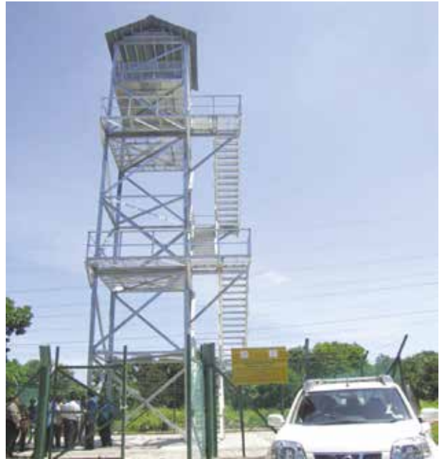
Pembinaan menara tinjau di Penur, Kuantan, Pahang Construction of watch tower in Penur, Kuantan, Pahang
