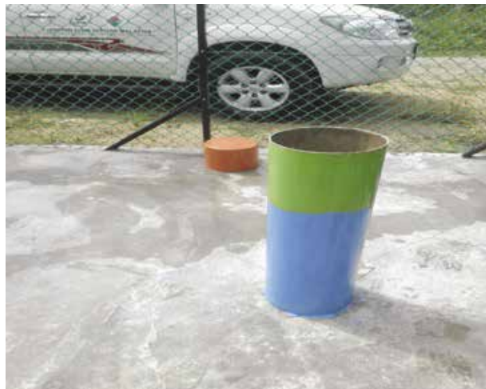
Telaga Air Tanah di Bachok, Kelantan Tube Well Constructed in Bachok, Kelantan
