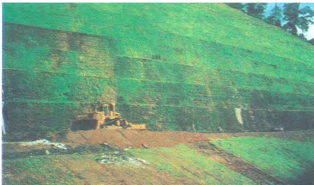
Erosion Prevention and Control Measures: Terracing /Benching
