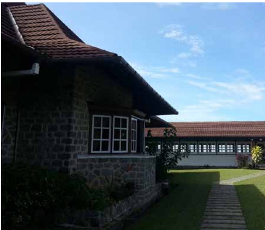
Figure 1: Low embodied energy building (bungalow, Fraser's Hill)
