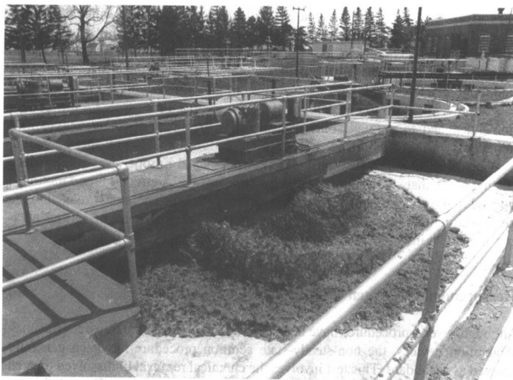
FIGURE 5.16 Low-speed surface aerator.
