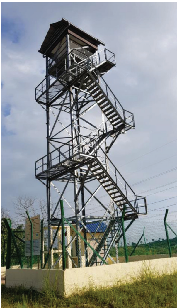
Menara tinjau di Kuantan, Pahang Watch tower in Kuantan, Pahang
