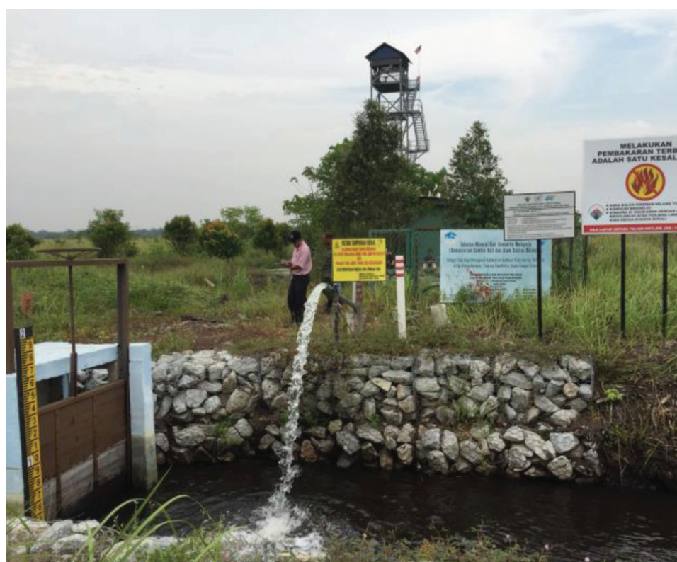
Kombinasi menara tinjau, telaga air tanah, sekatan saluran dan papan tanda larangan pembakaran terbuka di Kuala Langat, Selangor Combination of tube well. Check dam, watch tower and open burning prohibited sign at Kuala Langat, Selangor
