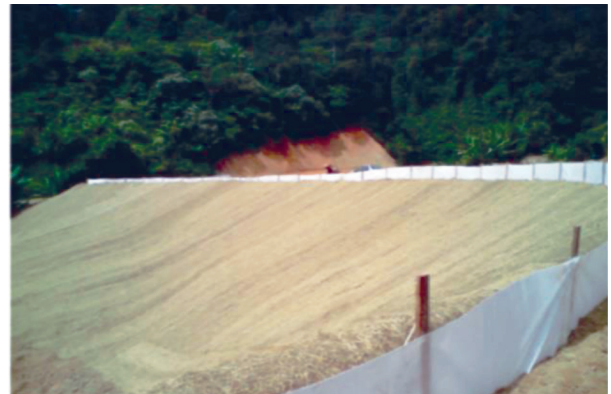
Silt Fence Silt Fence
