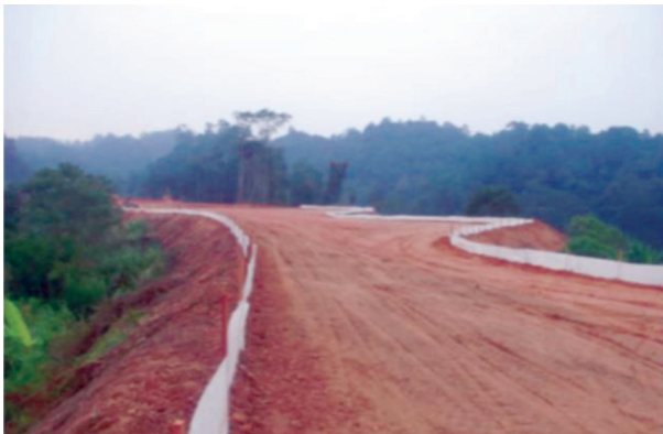
Silt Fence Silt Fence
