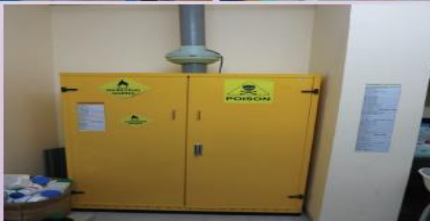
Figure 7: Chemical storage area
