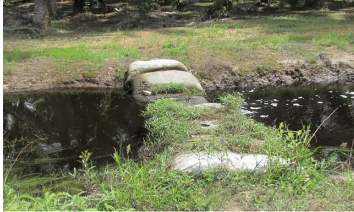
Gambar 4.7 : Check Dam Geobag
