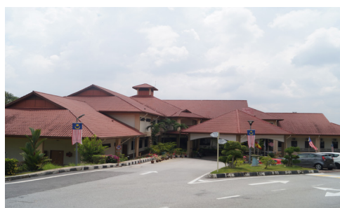
EiMAS Building, Bangi, Selangor
