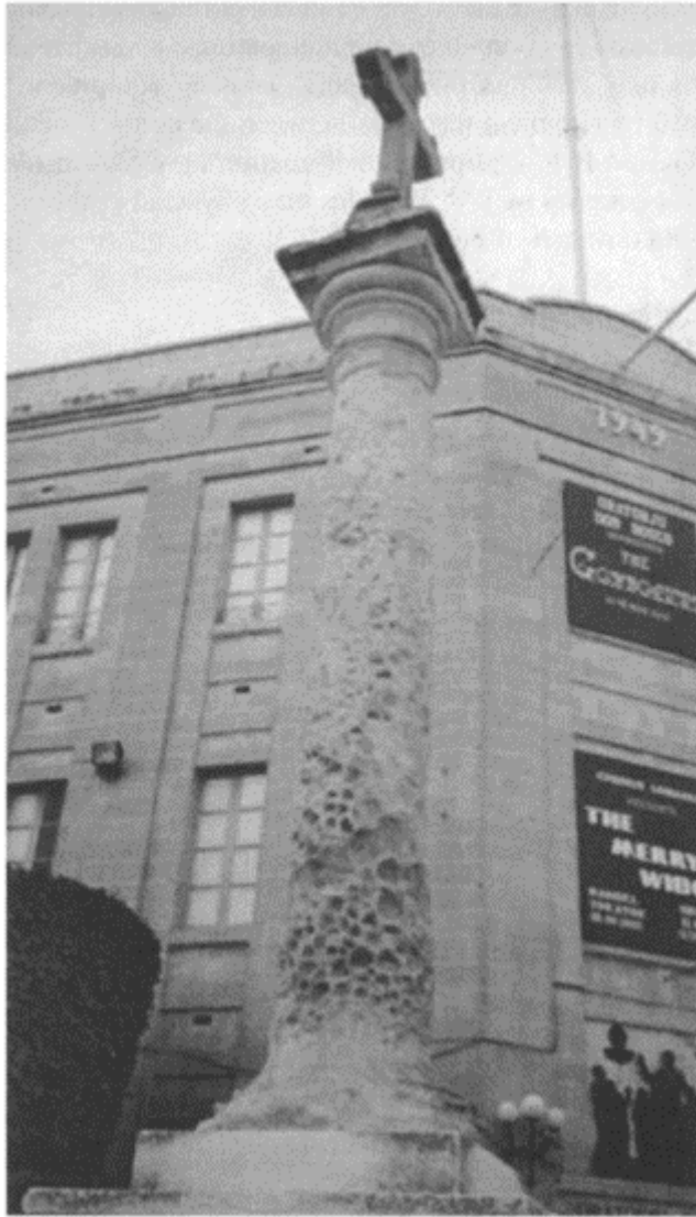
Figure 6.6 Erosion of carbonate column in Maltese square. (Courtesy of DHD Multimedia Gallery, http://aj.hd.org/ .)
