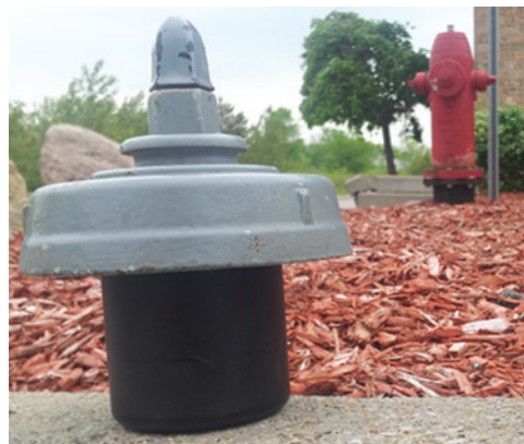
Figure 9.5.3 Echologics CAM unit is placed inside the hydrant cap with AMI communications (Source: David Hughes).
