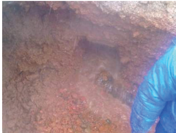
Figure 9.1.4 Leakage site excavation (Source: Đevad Koldžo).
