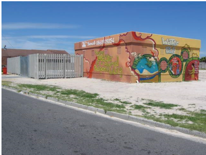
Figure 3.35 External view of the Mitchell's Plain installation.
