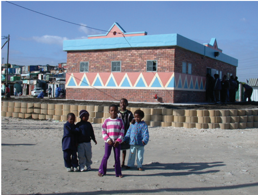
Figure 5.1 Initial Khayelitsha installation shortly after completion.
