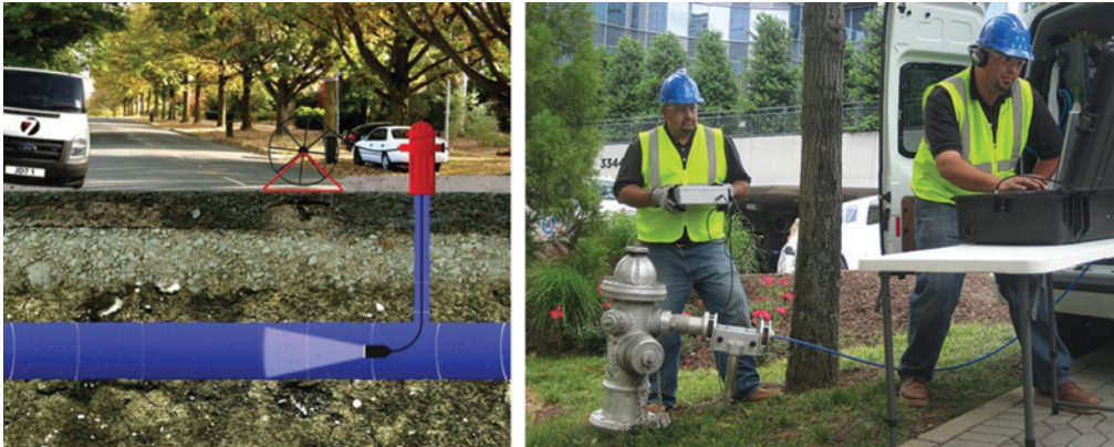
Figure 2.6 Push tethered system which can be operated with or against the water flow with access through tapping point or fire hydrant (Source: JD7).
