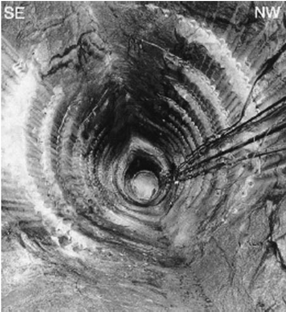
Fig. 5.10 Failed tunnel in the Canadian URL caused by high primary rock stresses [1]
