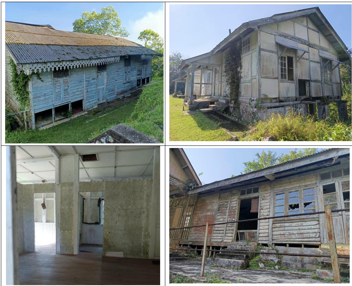
Figure 5.6 Some of the wooden buildings on the site to be demolished
