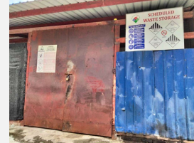
Proper Scheduled Waste Storage Area
